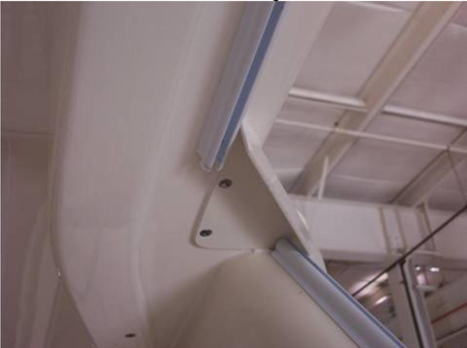
2. Once the 5' 6" track is secure add a 7' 6" pc to both ends. Track should extend around corner all the way to the arch style support. Trim ends of track 1in passed aluminum diverter on each side; keep the track tight to the diverter as shown in the picture.
